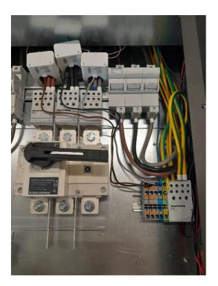
Mount the 5G2.5 mm<sup>2</sup> cable to the connecting block, respecting the colour assignment. The 5G2.5 mm<sup>2</sup> cable is secured with a 20A circuit breaker in the distribution panel.
