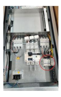
Phases 1, 2, 3 and neutral are directly connected to the fuses, while the ground is connected to the connector just right of the fuses.
