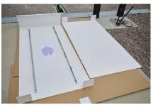
d. When assembling the EV Ultra anchor, a dummy top plate is used to determine the correct dimensions. This dummy plate has the correct dimensions, but not the correct solidity for the EV Ultra.
