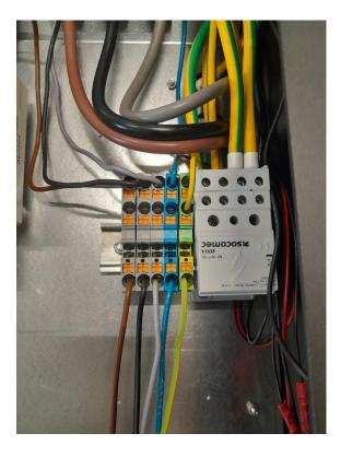
After removing the pre-wired cable and installation of the 5G 2.5 mm<sup>2</sup> cable, the installation of the power supply cables is the same as for a TN-C grid.
