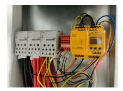
The remaining six control cables have a label from 1 to 6. Mount each cable to the corresponding connector within the EV Ultra. Use a small screwdriver to connect the cable.
