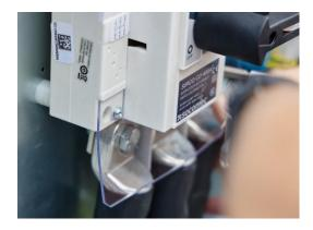
Connect the ground to the distribution block on the right of the EV Ultra, using an 8 mm hex wrench. Tighten it to **25 Nm**.
