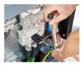
Protect the power supply cables using the plastic cover of the load break switch.
