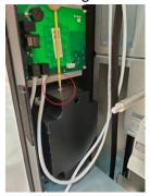
• When the desired tightness is achieved, tighten the set screw on the side of the cable holder. This makes sure the position of the top screw doesn't change when manipulating the charge cable.
