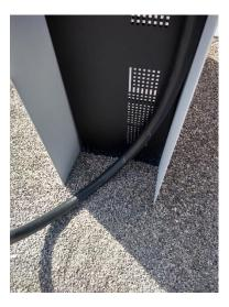
The EV Ultra can be placed maximum 3 cm below the top of the surrounding soil for aesthetic purposes. It cannot be placed lower as there will be risk of water ingress.
