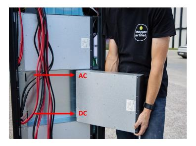
The inverter is into position when the right side of the inverter touches the right side of the slot.
