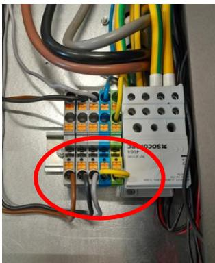
Use cable lugs M10 with a maximum width of 35 mm and connect phase 1, 2 and 3 to the load break switch. The screws should be tightened with a torque of **40 Nm**.
