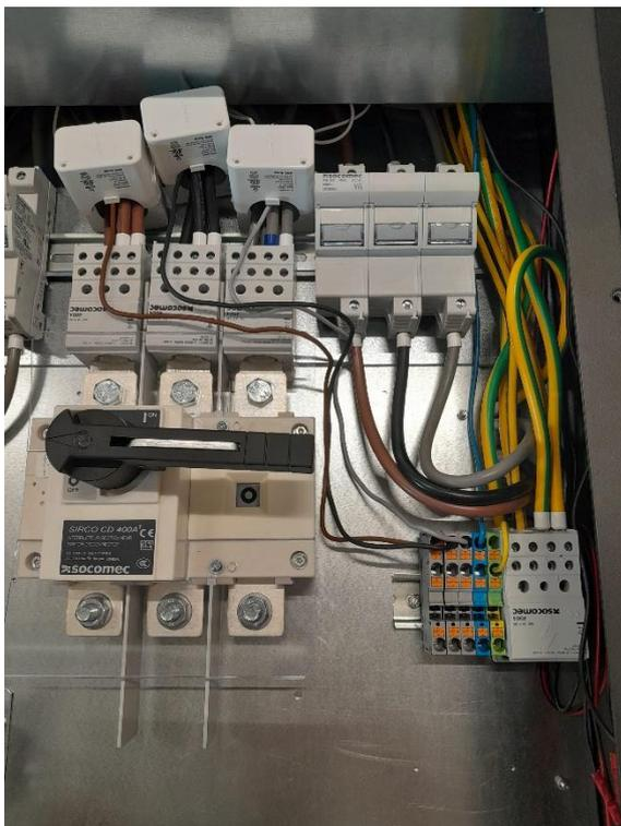
Mount the 5G2.5 mm<sup>2</sup> cable to the connecting block, respecting the colour assignment. The 5G2.5 mm<sup>2</sup> cable is secured with a 20A circuit breaker in the distribution panel.
